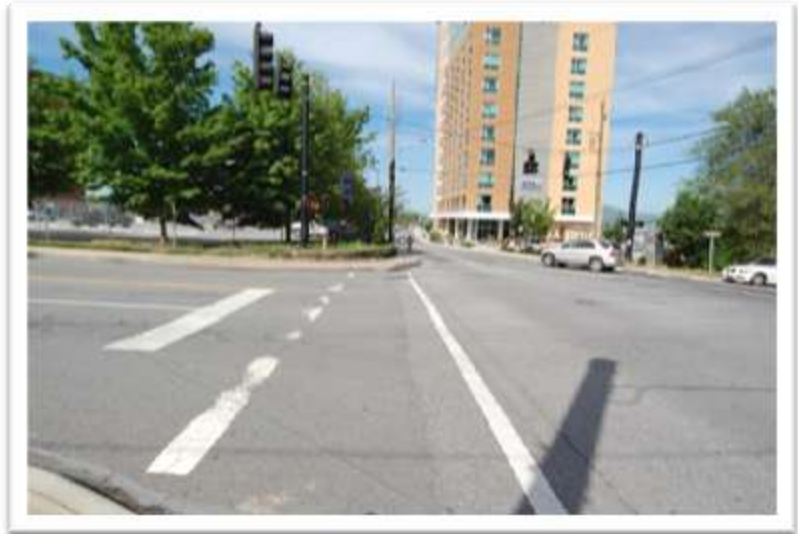
Location: Haywood St. & O'Henry Ave. Notes: Bushes on Northeast corner need trimming so they do not hide crosswalk lights. The Southwest corner lip needs smoothing.
